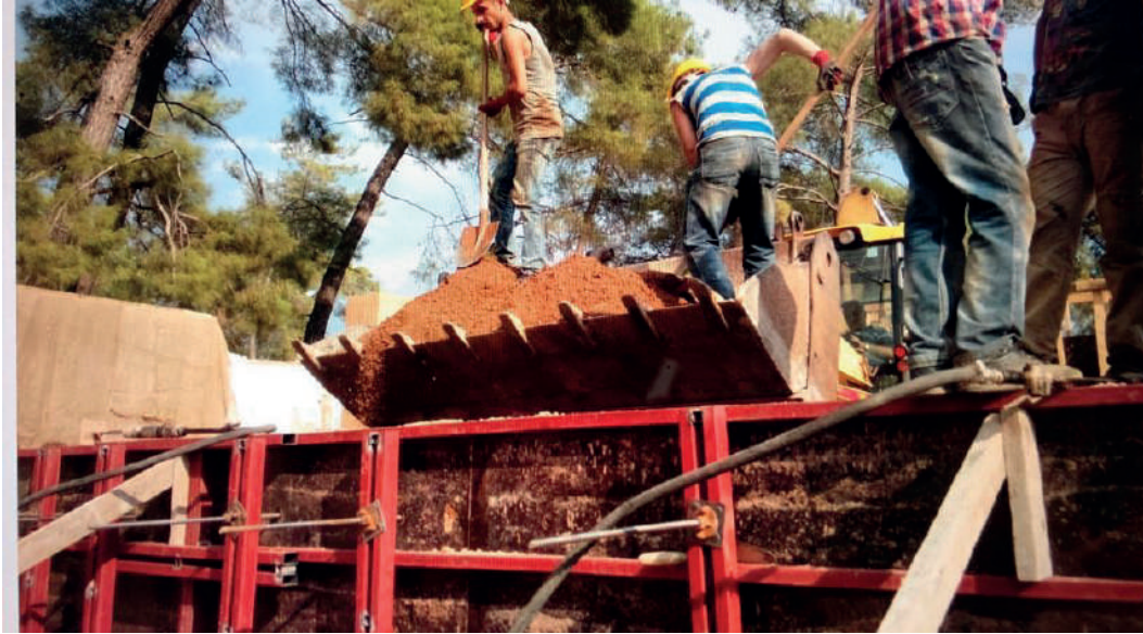
KEPÇE İLE DOLDURMA • FILLING WITH EXCAVATOR
