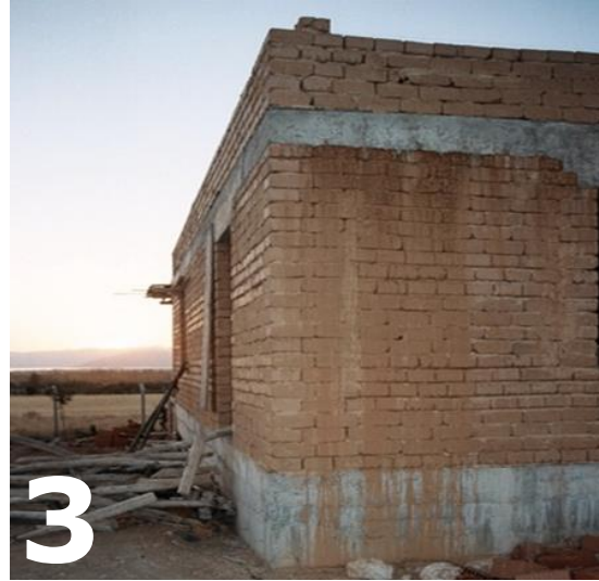
Earth construction without stabilization is damaged by water. (3)
