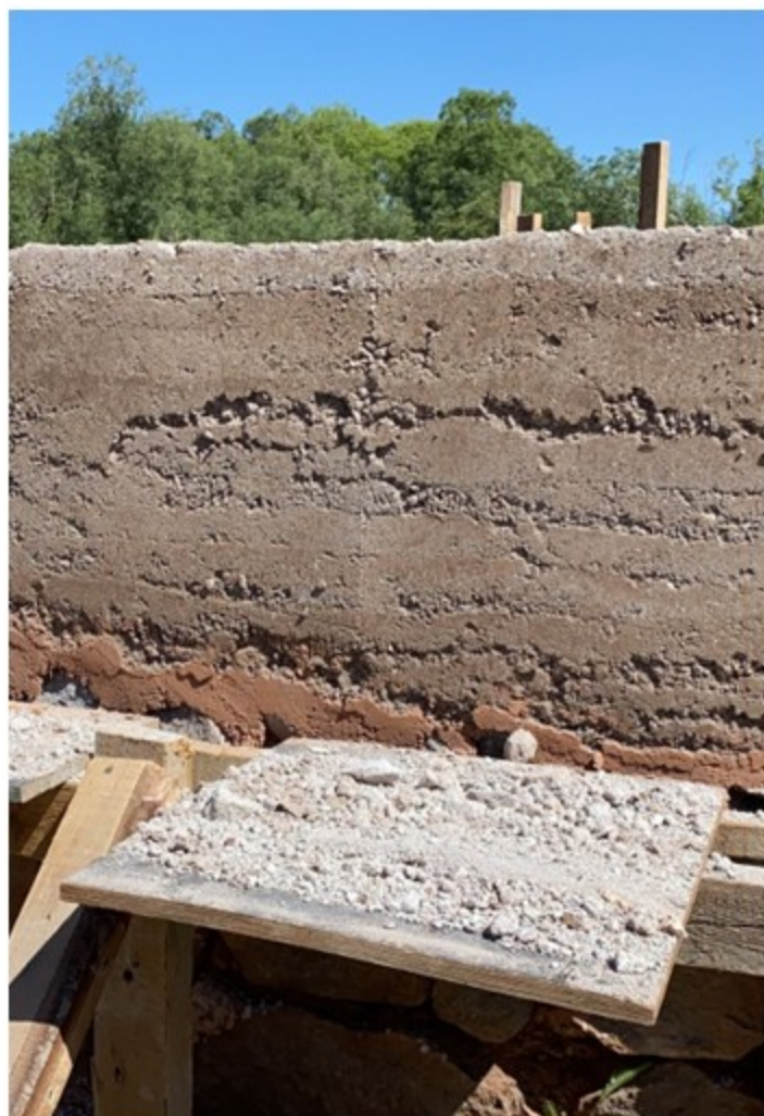
The first 60 cm of the two main earth walls were built, 10 June 2021
