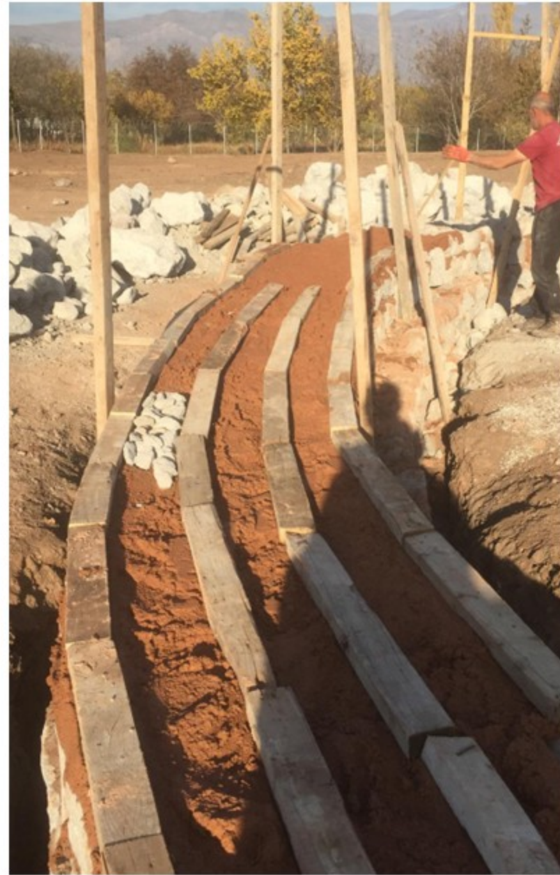
WOODEN BOND BEAMS
