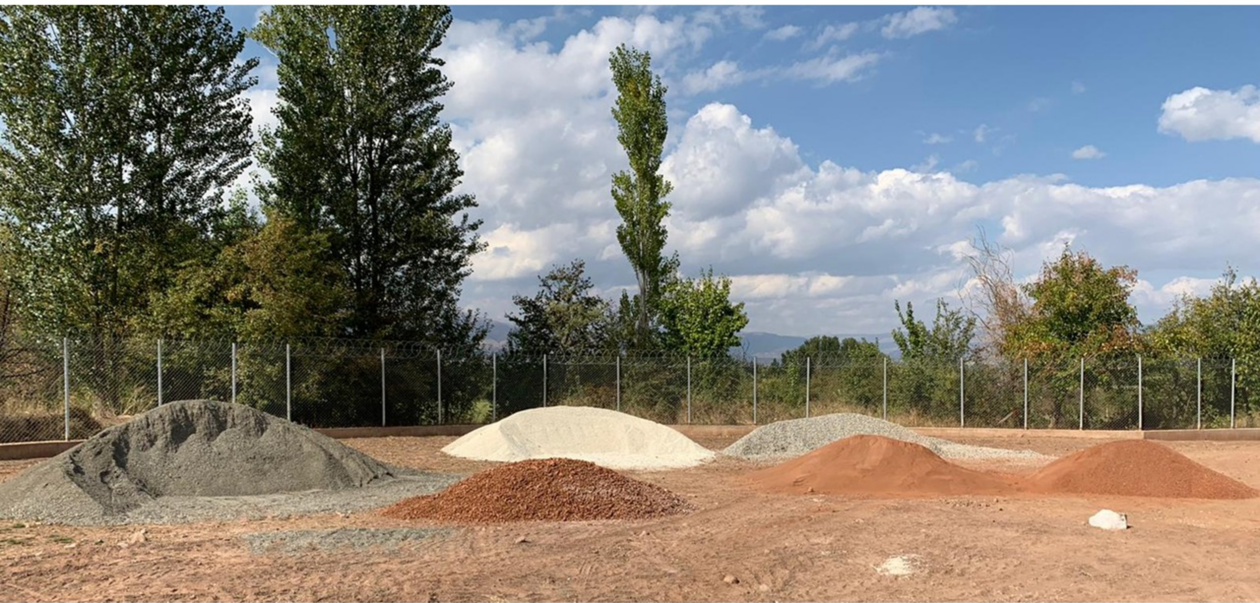
BLOCKAGE LAYER and KHORASAN MORTAR MATERIALS
