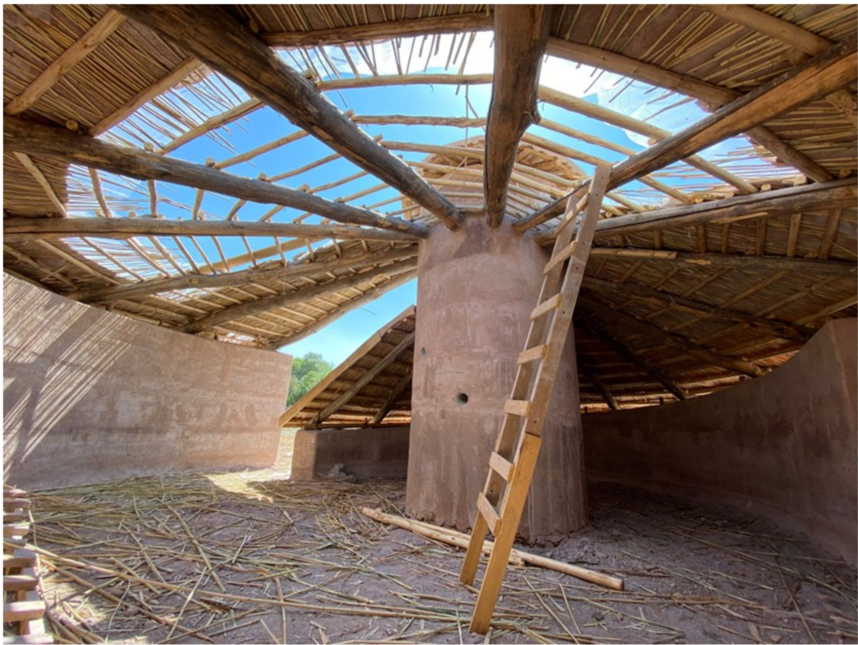
Layers visible during roofing, 31 August 2021
