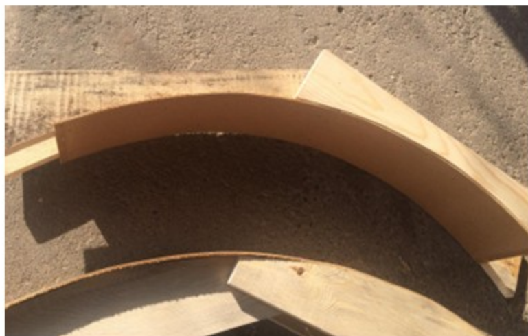
Wall molds made of plywood
