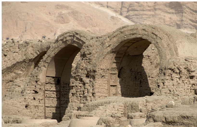
Figure 9. the silos' arches with four courses [10]
