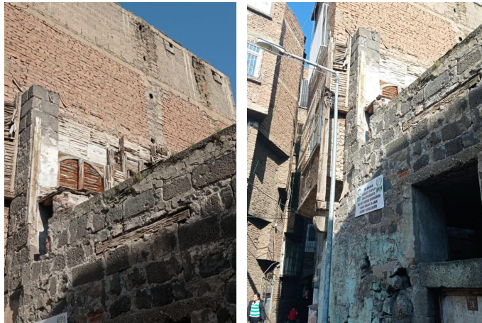
Picture 5. The exterior wall made with the Baghdadi construction technique in the Suriçi region of Diyarbakır
