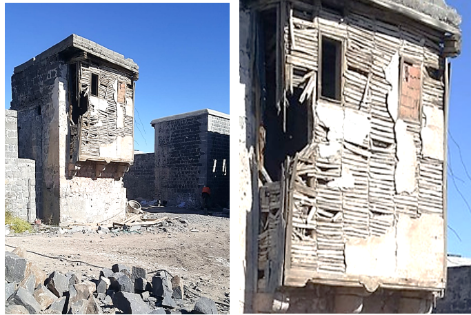
Picture 2. A bay window made with the bagdadi construction technique in the Suriçi region of Diyarbakır
