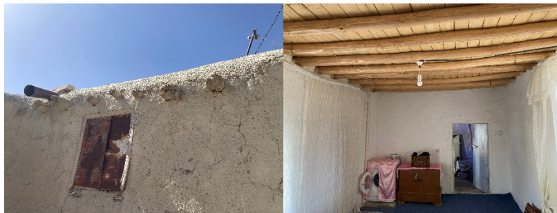
Figure 6. Exterior and interior view of the flat earthen roof from Mollatopuz Village (Gökdemir Archive)
