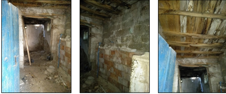
Figure 24. Structural damage observed in the bathroom section of Faik Bey Mansion (2023)
