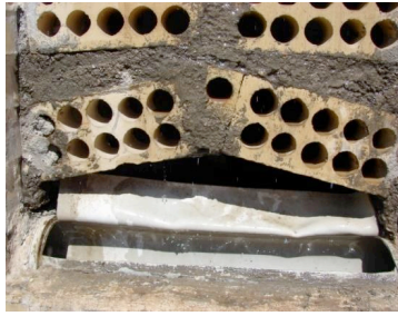
Figure 19. The gutter beneath the porous clay bricks facilitates the return of water to its source.
