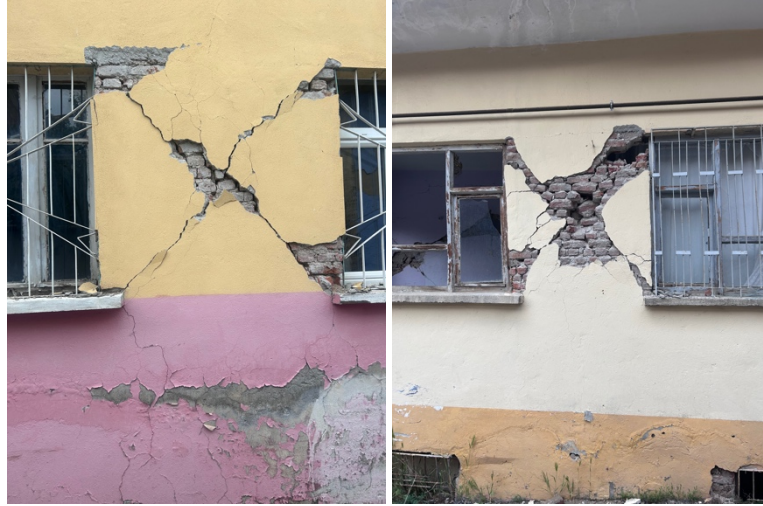
Figure 11. Examples of structural cracks [11]
