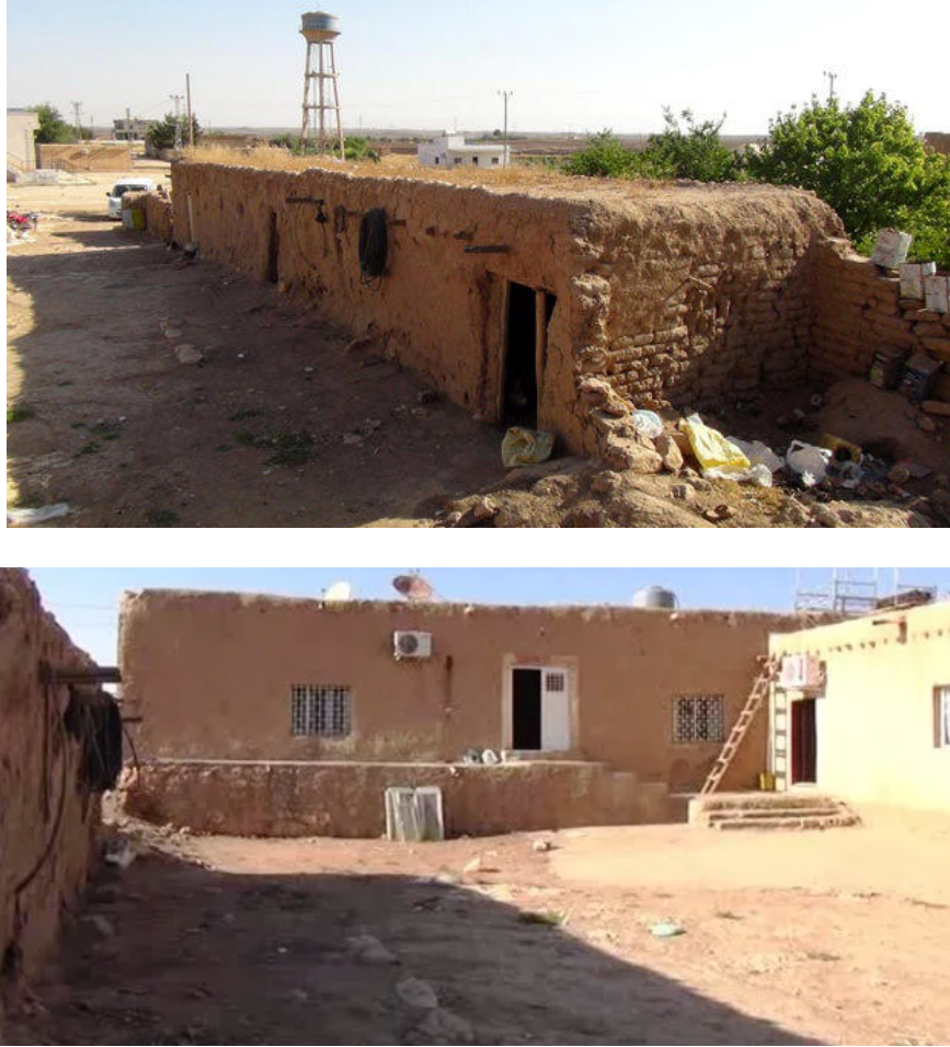
Figure 1. The adobe structure examples located in the Alakuş neighborhood of Kızıltepe, Mardin, exhibit issues such as 'cracks and deformations, warping and bending, and color changes' attributed to temperature differences.
