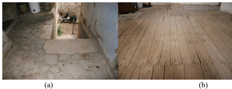
Fig.3.6. Upper floor slabs in Hüseyinik houses: (a) slate paving; (b) wood veneer
