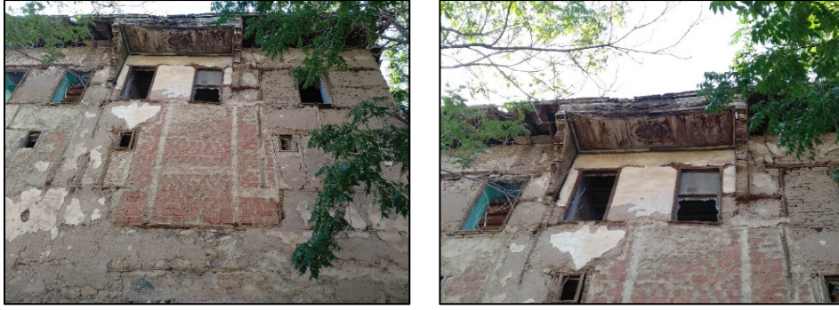
Figure 8. Structural damages observed on the southern facade of Faik Bey Mansion and the remains of the Köşk Room (2023)
