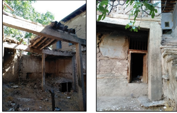
Figure 10. Structural damages and unqualified reinforced concrete annexes observed in the roof section of the Faik Bey Mansion courtyard (2023)
