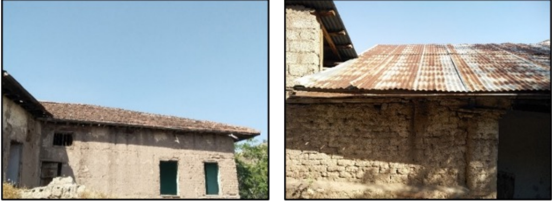
Figure 14. Faik Bey Mansion's non-original roof application and its structural damages (2023)
