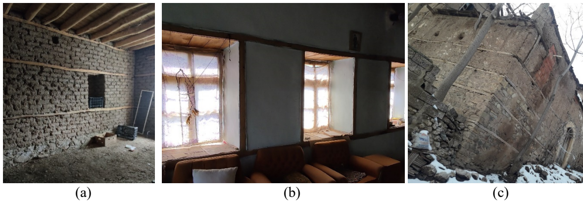
Figure 3.4. The use of beams and lintels in traditional Hüseyinik houses (a: intermediate beams on the inner wall; b: lintels on the windows; c: beams on the outer wall)
