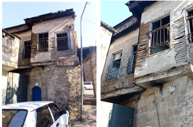
Picture 3. A bay window made with the bagdadi construction technique in the Suriçi region of Diyarbakır
