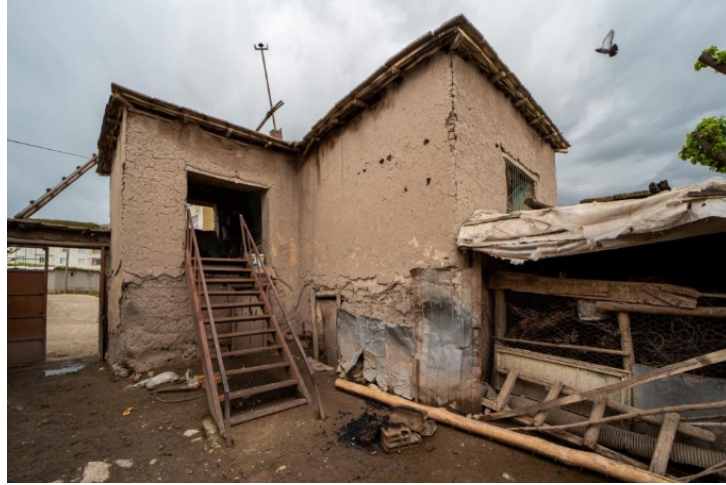
Figure 2. In the adobe structure example located in Diyarbakır, issues such as 'cracks and deformations, warping and bending, and color changes' have been identified due to temperature differences.
