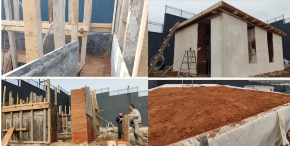
Figure 4: Temporary shelter plan and 4-module system produced from earth
