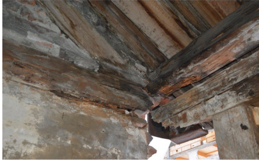
Figure 2. All of the geometric envelopes of the 175-year-old residential house are affected due to the micro-meteorological reversal of the vapour permeability and the following change of the dew point. (Source: Author)
