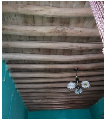
Fig.3.7. Beaming system (cisir) in Hüseyinik houses
