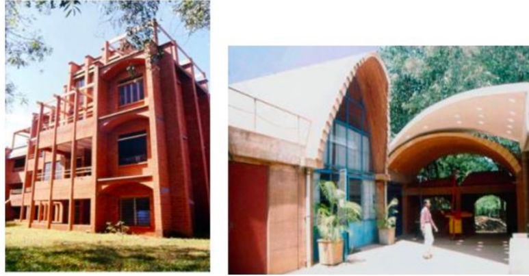
Figure 6. The example of integrated quarries by AVEI and the Auroville Earth Institute on the left was built entirely with stabilized soil (URL 9)
