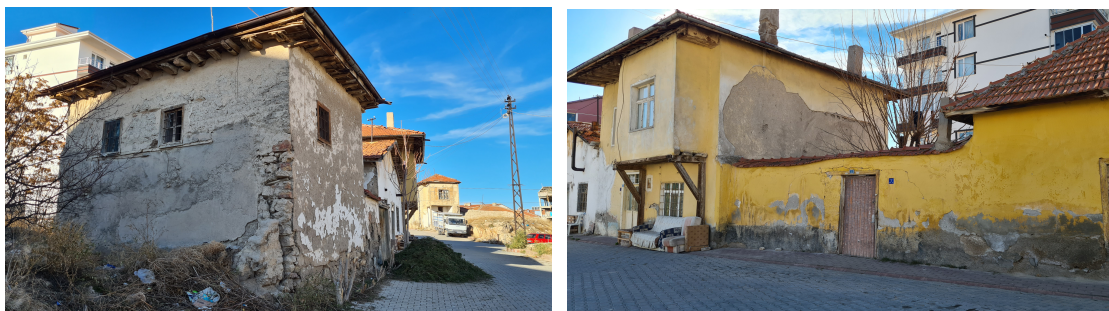
Figure 4. Erosion and plaster repairs on body walls (Author's Archive)
