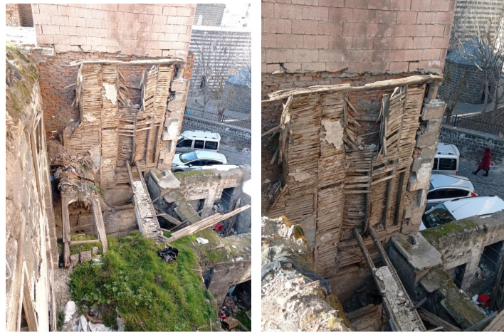
Picture 4. The exterior wall made with the Baghdadi construction technique in the Suriçi region of Diyarbakır
