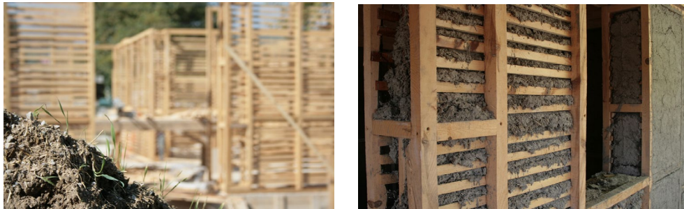
Figure 7-8. The adobe, which is not considered to be of high quality, was placed on the top with a shovel and compression provided by its own weight was ensured.
