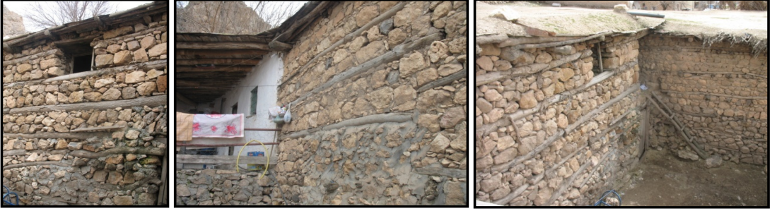
Figure.15. Use of bonding timber in walls (Diyarbakır-Silvan-Boyunlu Village)
