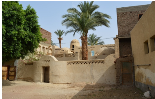
Figure 4. A house facade in the new village of Qurna village- Hassan Fathi - Luxor – Egypt, Taken by the Author
