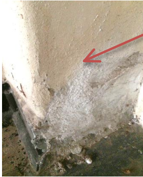
Figure 7. The ground water affection on an Adobe wall
