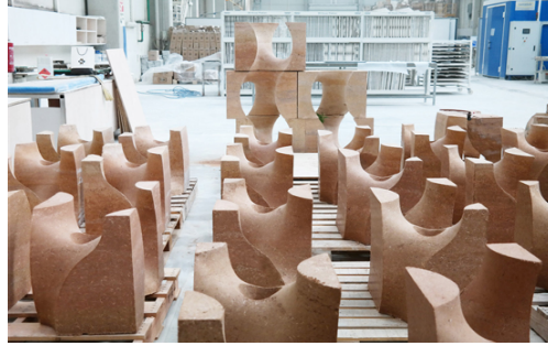
Figure 7. Fabrication of the blocks at Fibrobeton Facade Company Factory at Düzce.
