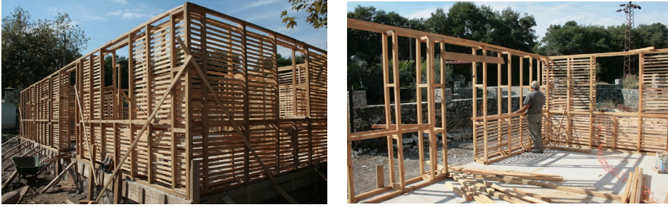
Figure 3-4. Corner Wooden Column (30 cm x30 cm.) Wooden Panels and Bagdadi Slats View
