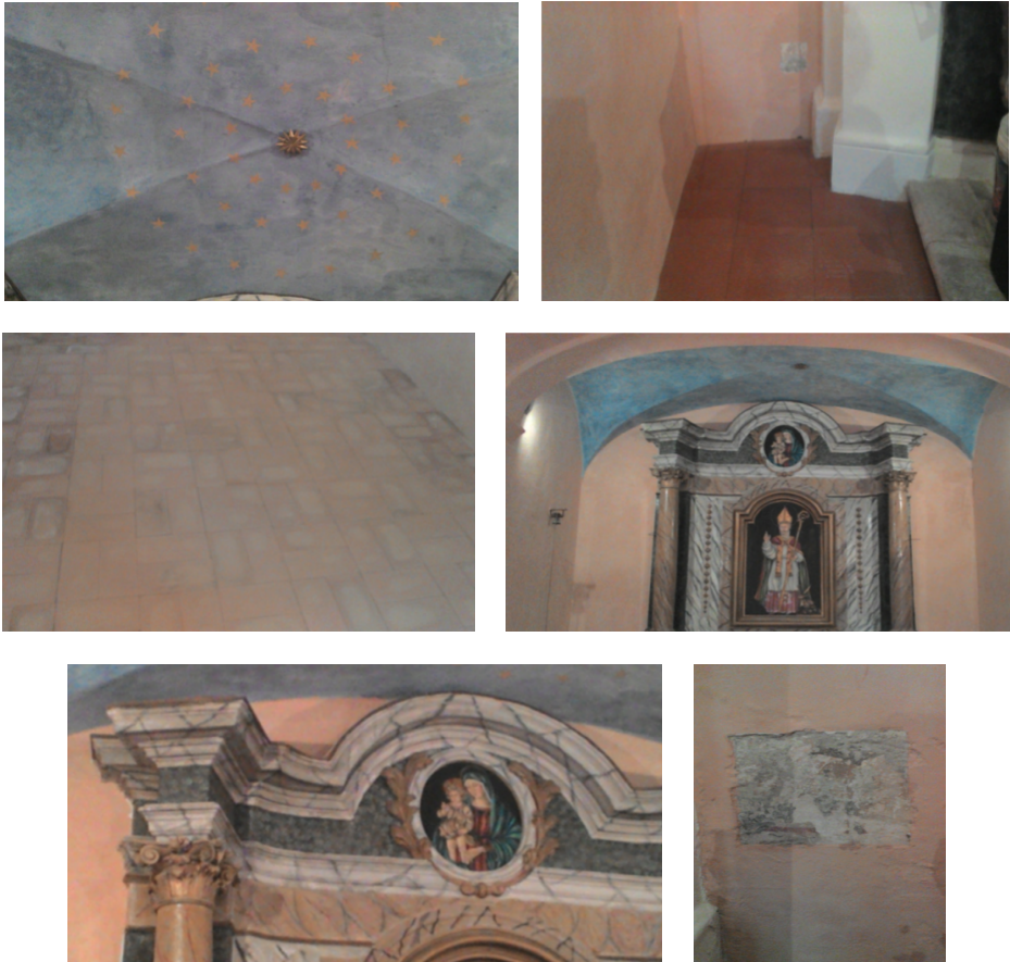
Figure 18-23. The final aspect of the restoration
