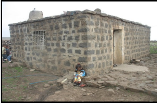
Figure.3. Pitch-faced use of stone (Diyarbakır- Hacı Koç Village)
