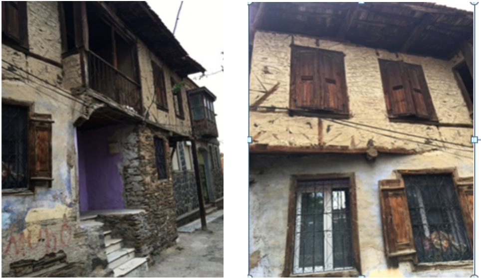
Figure 29. 30. Traditional Carcass Kula Houses with mortar surface
