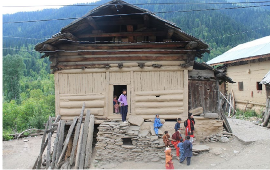
Figure 6: Picture describing elevated entry to the house (Upper Taobat Village)
