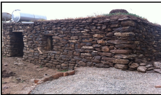
Figure.5. Stone wall – Dry bond (Diyarbakır- Karakoyun Village)
