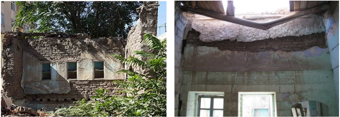
Figure 1, 2. Adobe houses in the Surici of Diyarbakır
