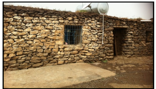
Figure.5. Stone wall – Dry bond (Diyarbakır- Karakoyun Village)
