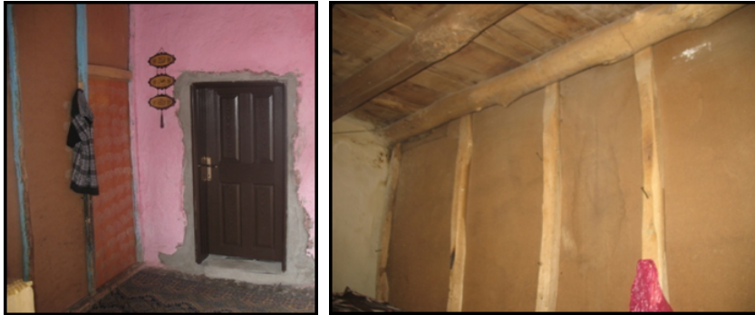
Figure 20. Use of wood as a partition wall (Diyarbakır - Silvan Boyunlu Village)
