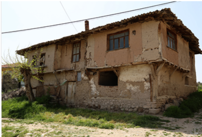
Figure 7. Mixed structural system
