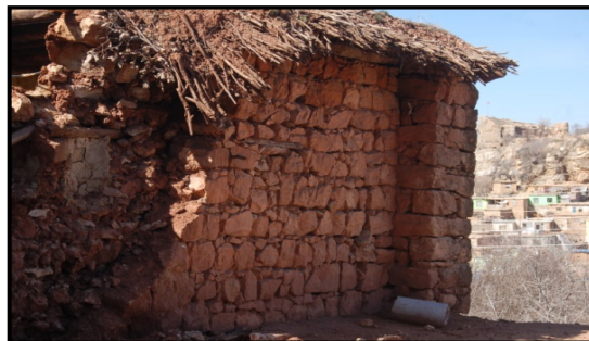
Figure.6. Stone wall – clay mortar (Diyarbakır- Silvan-Boyunlu Village)
