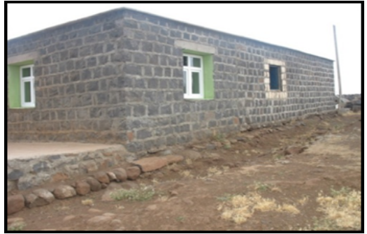
Figure.3. Pitch-faced use of stone (Diyarbakır- Hacı Koç Village)
