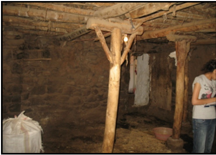
Figure 16. Wooden beam construction in stables
