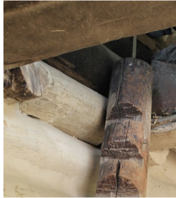
Figure 18: Wooden ladder access to attic level
