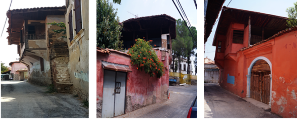
Fig 8. Example of the hayat seki and başoda projecting out into the street.
