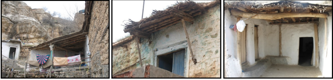
Figure 19. Use of wood as an eaves element (Diyarbakır - Silvan Boyunlu Village)
