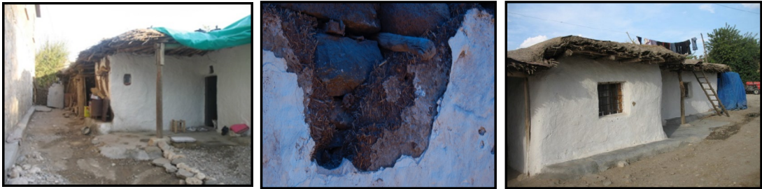
Figure.10. Use of lime on soil plaster in adobe constructions (Diyarbakır-Akdere Village)
