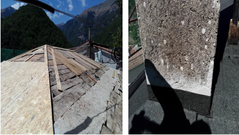
Figure 5, 6. Conservation of the roof and waterproofing
