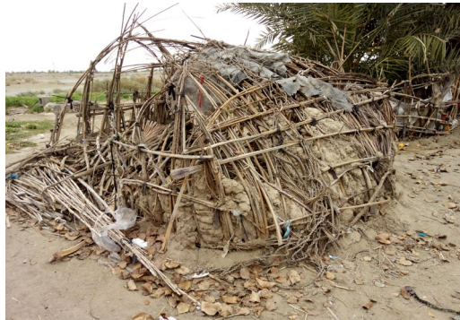
Figure 10. An example of kapar that was destroyed after 25 years (Credits: Bakhshi, 2019).
