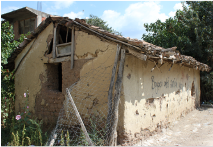
Figure 5. A barn with load bearing system
