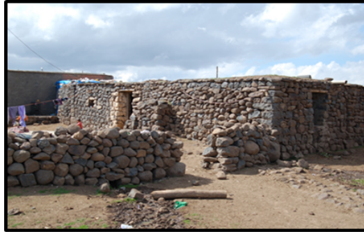
Figure 1. Basalt use as building material (Diyarbakır-Hacı Koç Village)
