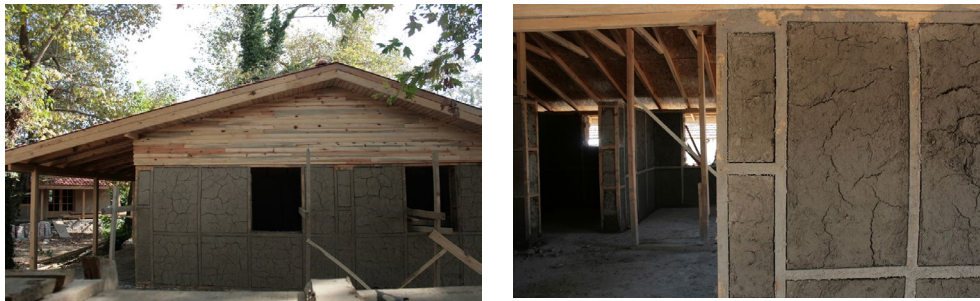
Figure 9-10. The gap formed on the surface of bagdadi slats is filled with the same material. All adobe surfaces and shrinkage cracks, except the wooden frame surrounding the panels, were plastered with earthen plaster.
