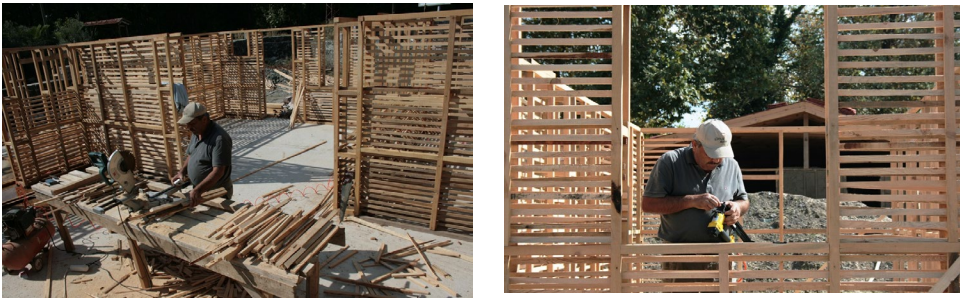
Figure 5- 6. Preparation of Bagdadi Slats and Nailing with Pressure Nail Gun in Place
