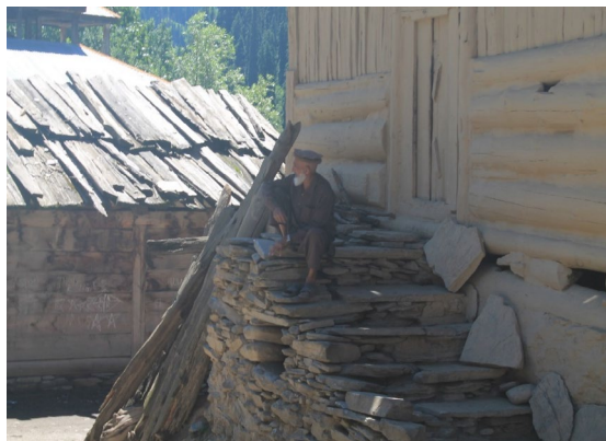
Figure 16: Outer Mud Insulated Walls
