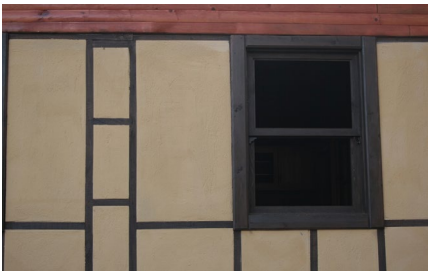
Figure 15-16. Water-based Paint on The Facade
