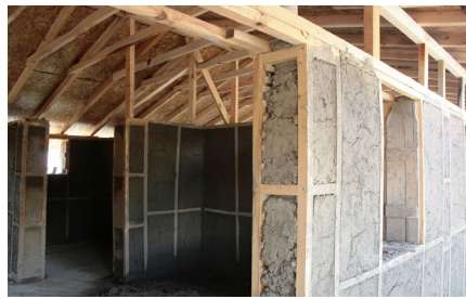
Figure 13-14. Wooden Roof Over The Upper Wooden Beams Surrounding the Building.
