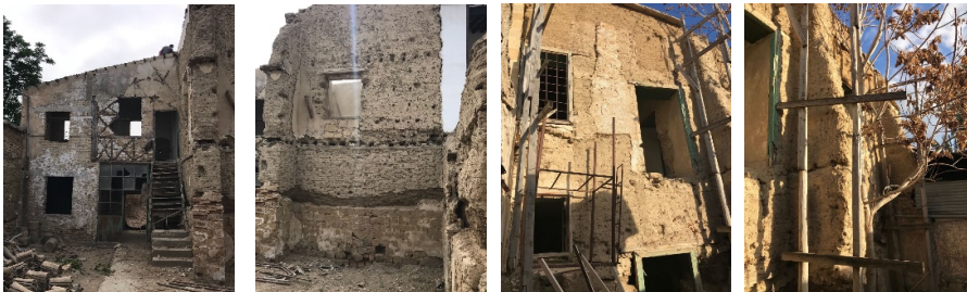
Figure 4. Part added to the original structure
