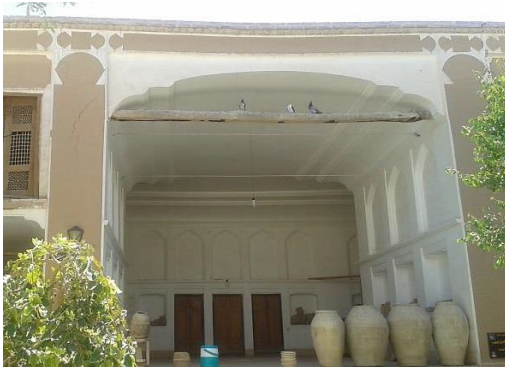
Figure 4. Vernacular solutions: application of wooden tie beam in Yazd, Iran (left image) (1); application of buttresses in the Andean region (right image) (9).
