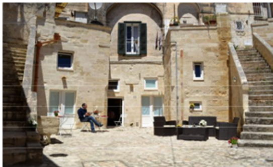
Figure 9. The neighborhood of Ancient Convicino on the side overlooking the small square after rehabilitation.
