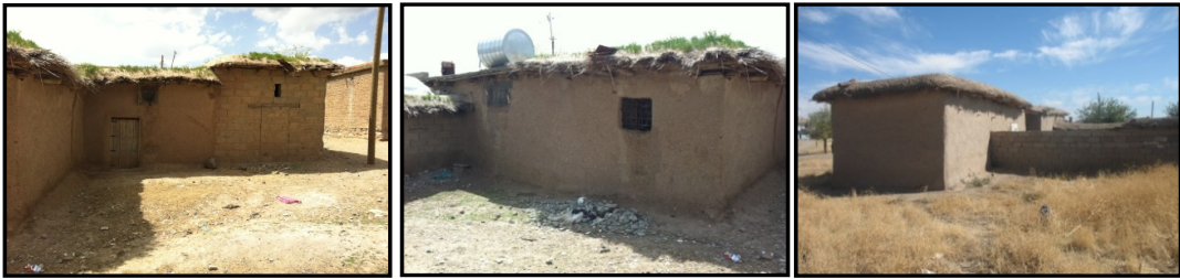
Figure.14. Cover coat type – Earth-covered roof (Diyarbakır Sumaklı Village /Diyarbakır-Bismil-Erler Village)
