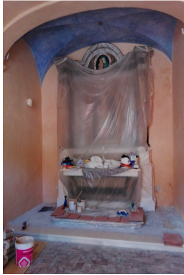
Figure 10. Protection of the altar restored during the work of the church
