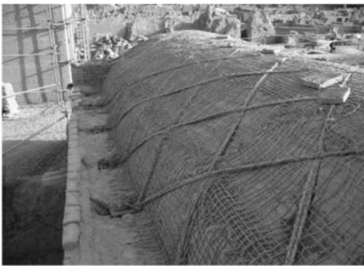
Figure 5. Strengthening a vaulted roof with mesh made from palm-fiber, Bam citadel, Iran (10).
