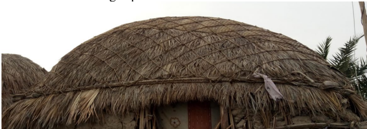
Figure 7. Roof structure system (Credits: Bakhshi 2019).
