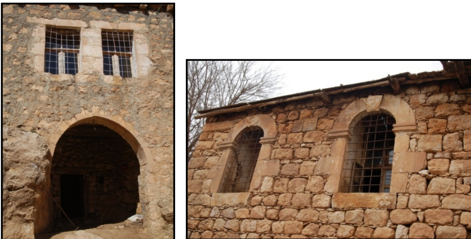
Figure.8. An example for the use of arches at the door and windows (Diyarbakır-Boyunlu Village)
