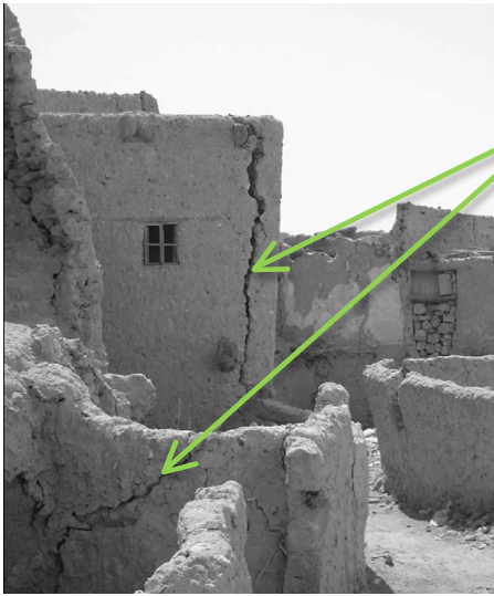
Figure 10. The cracks in the wall, Siwa, Egypt
