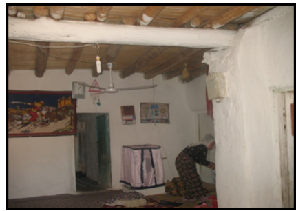
Figure 17. Wooden beam construction in housing units
