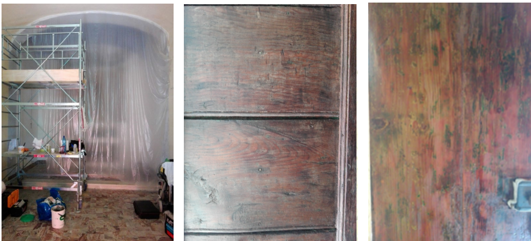
Figure 7, 8, 9. Protection of the altar, restoration of the inner and outer part of the door
