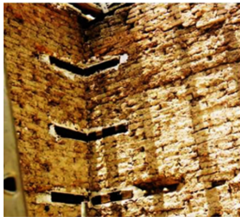
Figure 11. Installation of timber beams for the treatment of a vertical discontinuity
