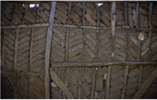
Figure 6a. Wooden framework with diagonal.. Figure 6b. ..with horizontal adobe block fillings
