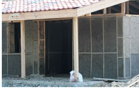
Figure 12. Wall Exterior View
