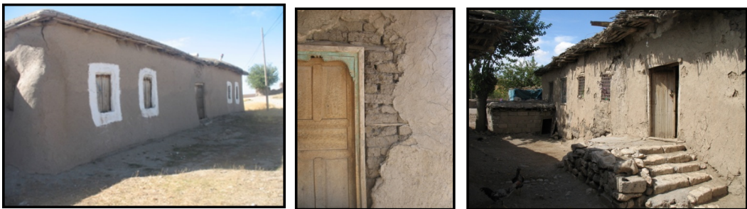
Figure 9. Use of soil plaster in adobe constructions (Diyarbakır - Akdere Village, Erler Village)
