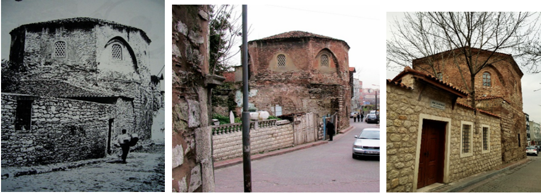
Figure 22-23-24. The condition of wall; in original, during the 20th century and after the restoration.
