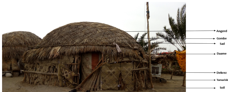
Figure 3. Local construction materials, ShahrDeraz (Credits:Bakhshi, 2019)
