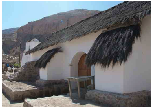
Figure 4. Vernacular solutions: application of wooden tie beam in Yazd, Iran (left image) (1); application of buttresses in the Andean region (right image) (9).
