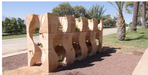
Figure 2. Common-action Walls, a sustainable rammed-earth wall that performs as a vertic garden wall
