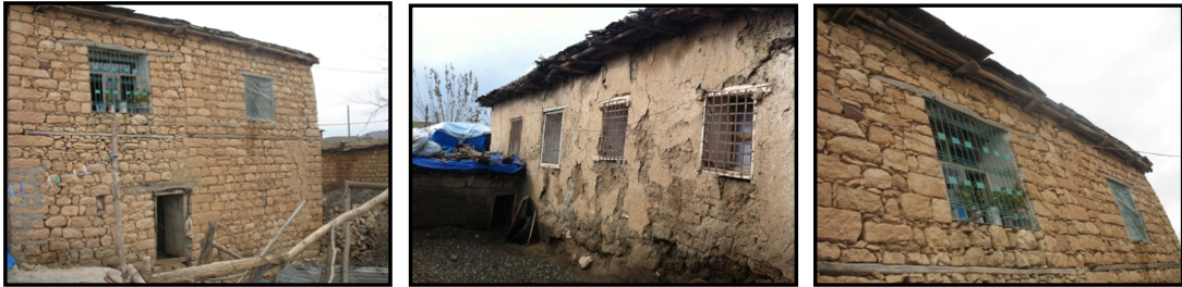
Figure.11. Use of bonding timber at windows (Diyarbakır-Akdere Village, Boyunlu Village)
