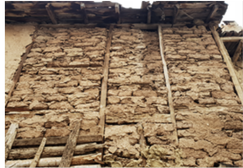
Figure 6a. Wooden framework with diagonal.. Figure 6b. ..with horizontal adobe block fillings
