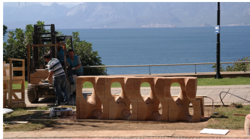
Figure 11. On-site application of Common-action Walls at Karalioğlu Park, Antalya,for IABA 2017.
