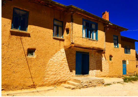
Figure 1. The earth based patterns around the main entrance door (Source: Cüneyd Ülvan Archive)
