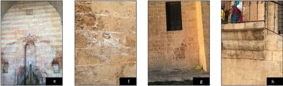
Figure 4. Chemical distortions seen at Kasımiye Madrasa
