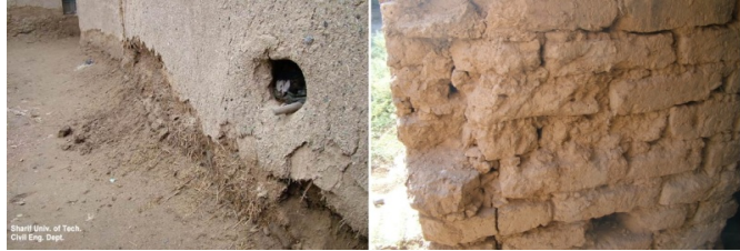
Figure 7. The ground water affection on an Adobe wall
