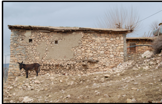
Figure. 2. Limestone as a building material (Diyarbakır-Boyunlu Village)
