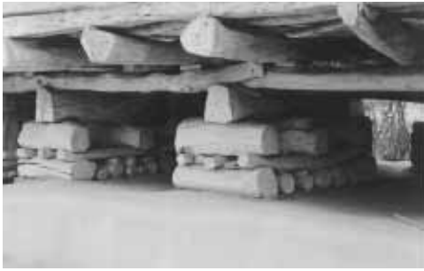
Figure 3. Vernacular solutions: application of seismic base isolation in Lahijan, Iran (left image) (7); Chinnneh wall after the Bam earthquake with slight damage (right image) (8).
