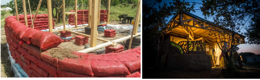
Figure 1. (a) Bathroom building exterior walls made of earthbags, (b) Bathroom building exterior (URL[3]).
