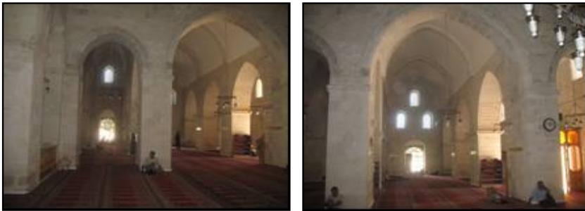
Figure 4. The arches on which the dome rests
