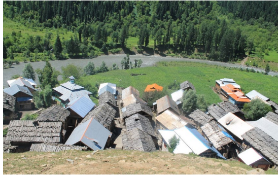
Figure 20: Wooden roofs for better Insulation
