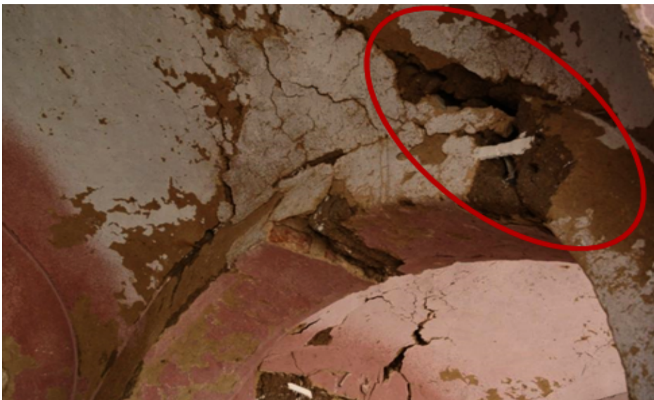
Figure 9. Adobe Disintegration, El.Qurna- Luxor, Egypt, Taken by author
