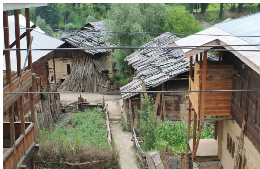
Figure 19: Washrooms are parasitic structures
