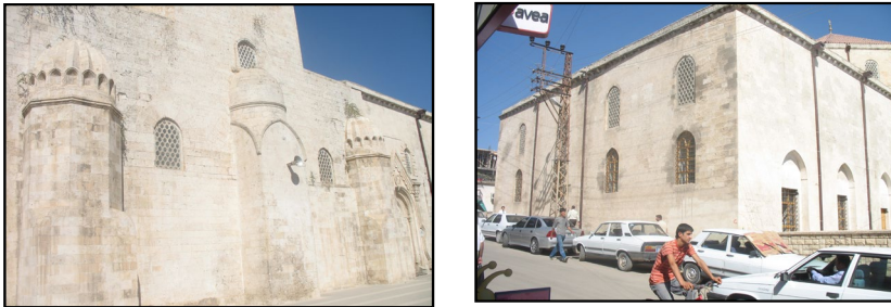
Figure 11. The buttresses at the Façade
