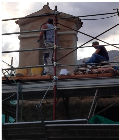
Figure 14. Restoration of the sailing bell tower
