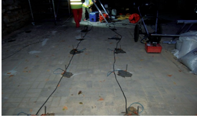
Figure 10. ERT implementation surrounding the building.
