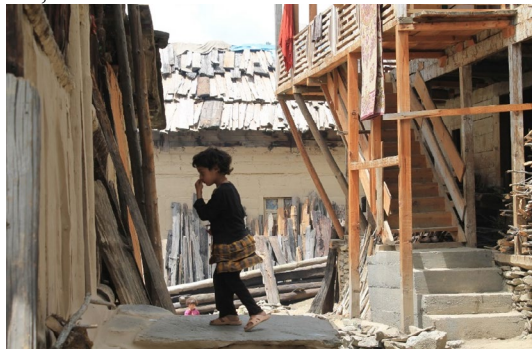
Figure 10: Access to the living area from Outside (Elevated entry)
