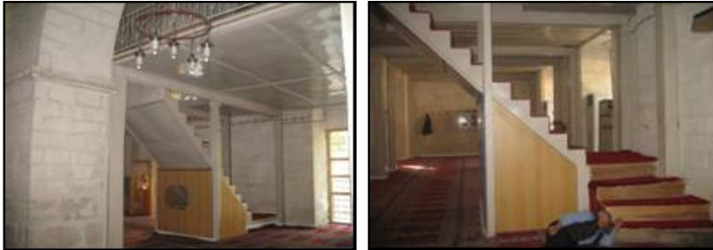
Figure 6. The Mezzanine Floor Later Integrated as Add-on and the Stairs that Provide Access to it
