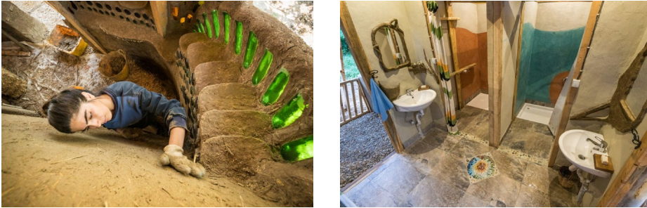
Figure 2. (a) Exterior walls are made of earthbags topped with cob bottle walls (b) Showers plastered with a colorful shiny tadelakt lime plaster (URL[3]).
