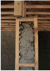
Figure 11. Wall Cross Section View
