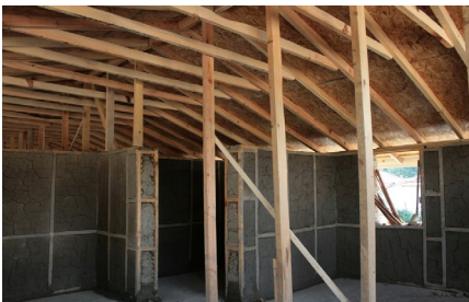
Figure 13-14. Wooden Roof Over The Upper Wooden Beams Surrounding the Building.
