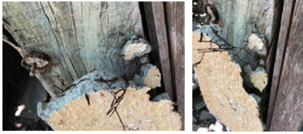
Figure 7 a, b. Soda pop caps used in nailing the plaster wire to the surface
