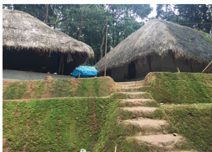
Figure 8a,8b. Image of dwelling 2 showing the structure(8a) and the plaster pattern (8b).
