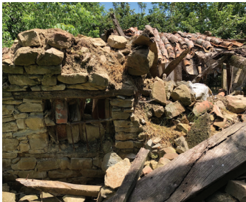
Figure 12 a. The stone wall of the building's rear façade
