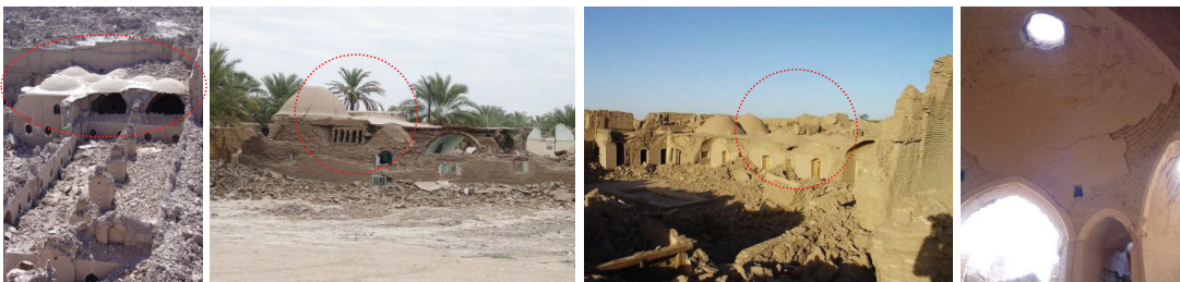
Figure 17,18,19,20. Remained earthen Domes in bam after earthquake (authors).
