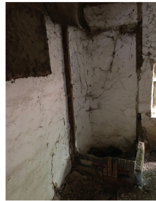
Figure 21 b. Remnants of a cabinet and shower unit in the Osman Ayvaz House
