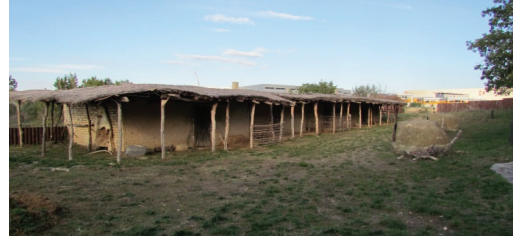
Figure 19. Aktopraklık Entrance of adobe houses Photo: Barancan Şahin
