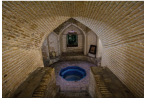
Figure 7. Sardab, Creation of evaporative cooling with the help of Qanat in Sardab. Generate thermal balance throughout the day using the Earth's thermal capacity.
