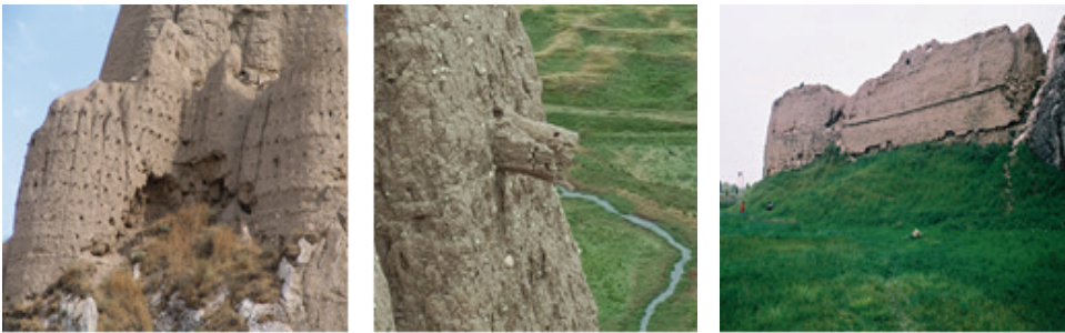
Photo 21, 23. Views of Wall and Tower with Bat Technique from Van Castle (Ş. Öztürk)
