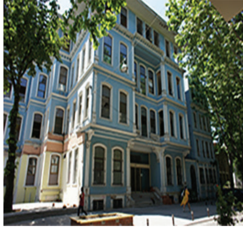
Figure 1. The building covered by the work located in Istanbul
