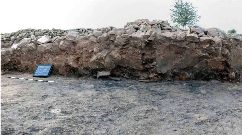
Figure 2. Vertical wooden beam slots from Trench 31 (TR31). The beams occurred at regular intervals along the wall's face, into which they were recessed. It is unclear if the lime plaster which otherwise covered the walls and floor of this room also covered the beams, or if they were left exposed.
