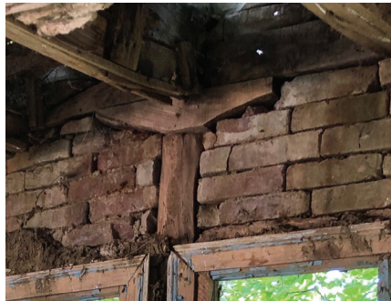
Figure 23 a, b. Lower and upper headings of support elements in wooden posts
