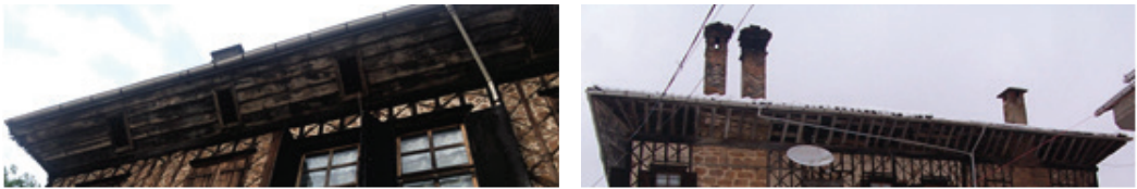
Figure 12. Balekoğlu Mansion Eaves Detail [F: E. Balık, 2019]
