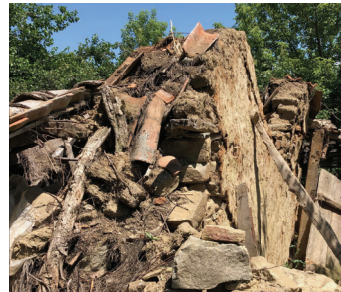
Figure 12 b. Stone masonry remnants of the side wall
