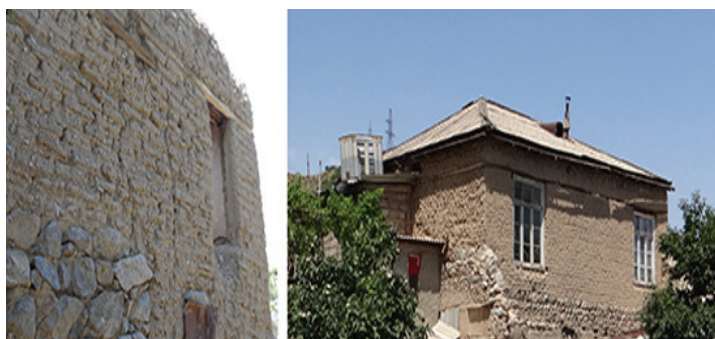
Figure 3. Residential building, build in mud brick and stone.
