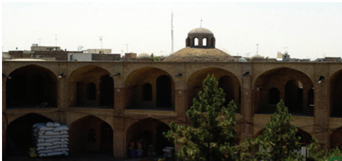
Figure 19. View of the Razavi Caravansaray [16]
