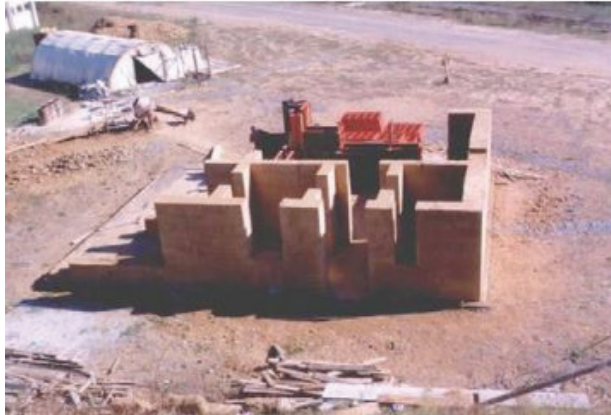
Figure 1 Aker building under construction[3]
