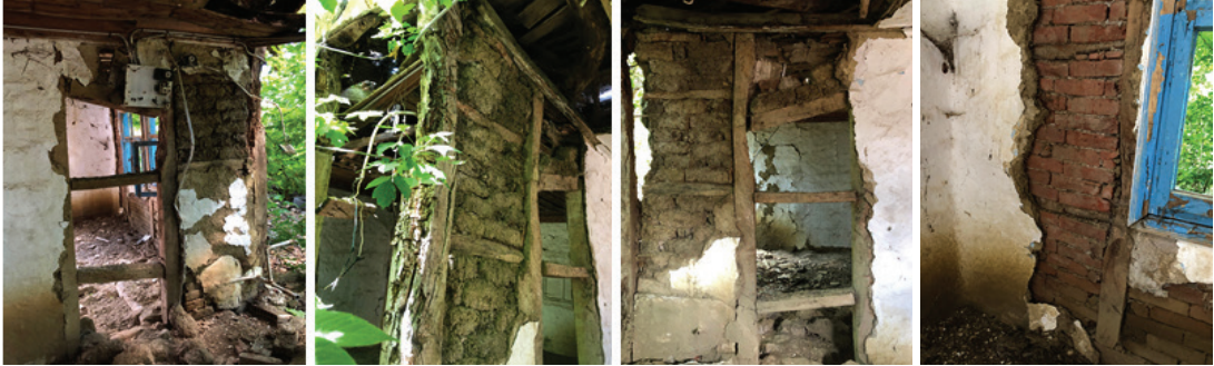
Figure 4 a. Mudbrick filled inner walls
