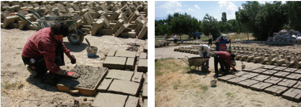
Photo 11, 12. Mud-Brick Preparation Views (Ş. Öztürk)
