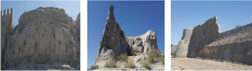
Photo 30, 32. Views of Wall And Tower With Bat Technique, Uzbekistan-Bukhara Castle (Ş. Öztürk)
