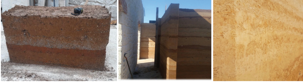
Figure 10. Wall samples from private building in Köyceğiz, Muğla, Turkey (Photo Credit by, Author)
