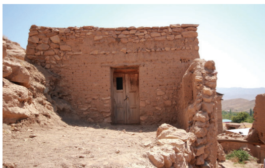
Figure 8 cottage before starting the workshop
