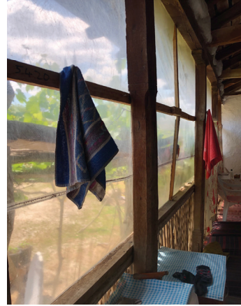
Figure 22 b. The Hüsniye Kökdemir House
