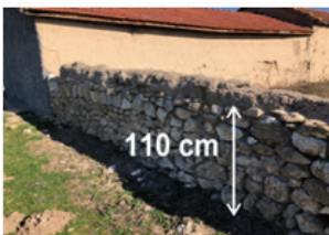
Figure 5 Stone foundation wall height level and wall width (2019).
