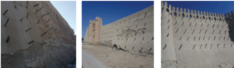
Photo 33,35. Views of Walls with Bat Technique, Uzbekistan-Bukhara Castle (Ş. Öztürk)
