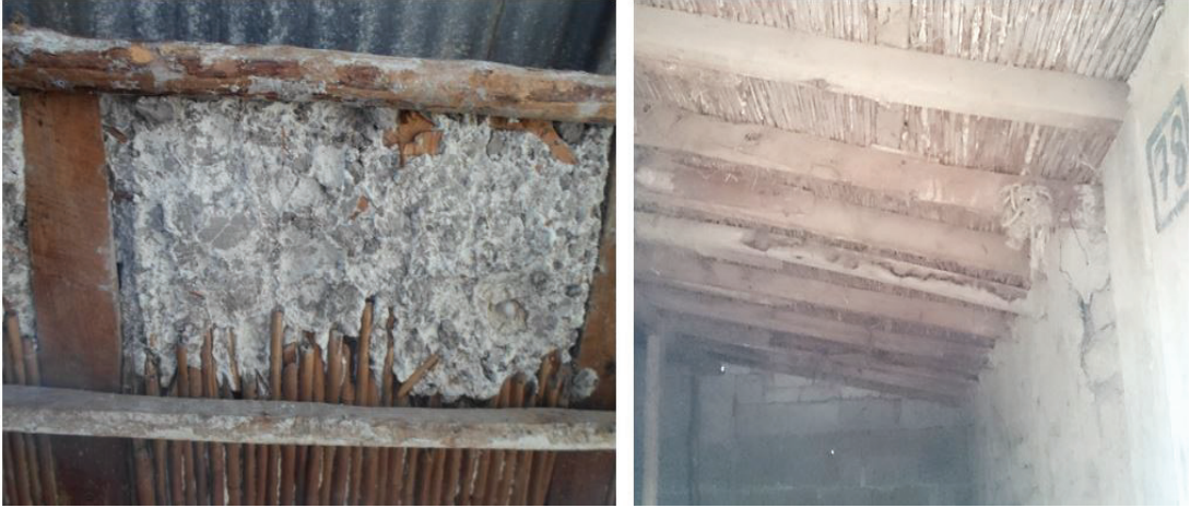
Figure 13: Muhacir Houses Dam Interior View [2]
