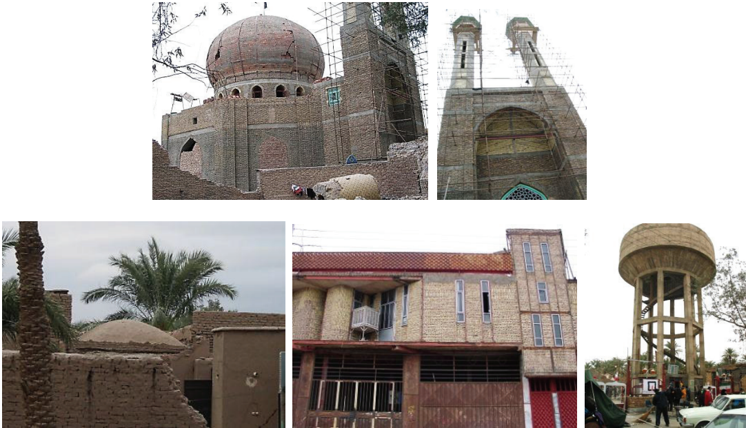
Figure 12,13. (below): The stability of Bam's jame mosque in earthquake (authors). Figure 14,15,16. (above): Remained buildings in bam's earthquake (authors).
