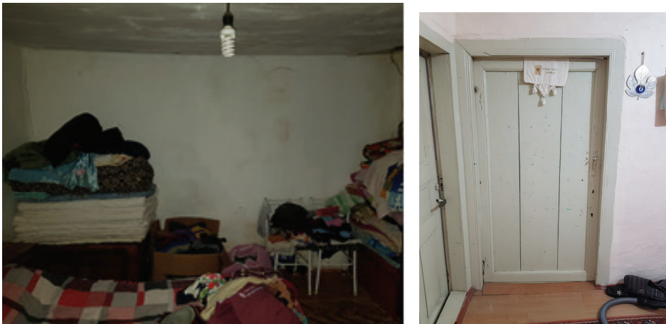
Figure 8. Mudbrick housing plasterboard ceiling and wooden interior doors.
