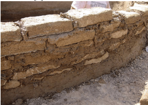
Figure 4,5. Examples of mudbrick walls of different thicknesses.
