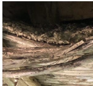
Figure 9 b. Earthen layer spread over sunflower stems
