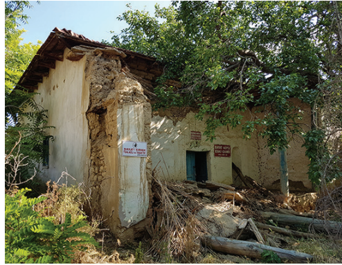
Figure 2. Bayat Mosque Entrance Facade View, 06 June 2019.
