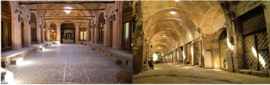
Figure 15. Bricked arches are seen in the bazaar [15]
