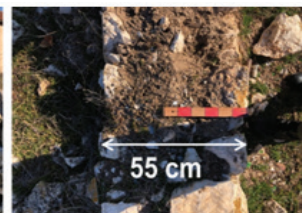
Figure 5 Stone foundation wall height level and wall width (2019).
