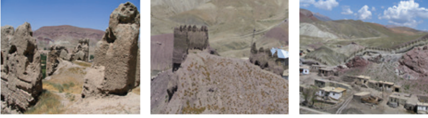
Photo 24, 26. Views of Walls and Towers with Bat Technique from Van-Hoşap Castle (Ş. Öztürk)
