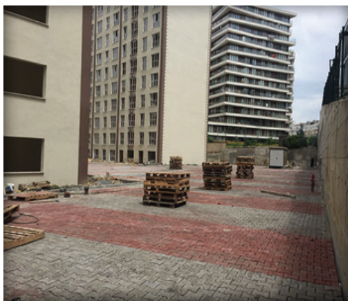
Figure 2. Reinforced concrete buildings from Istanbul, Turkey (Photo Credit by Author)
