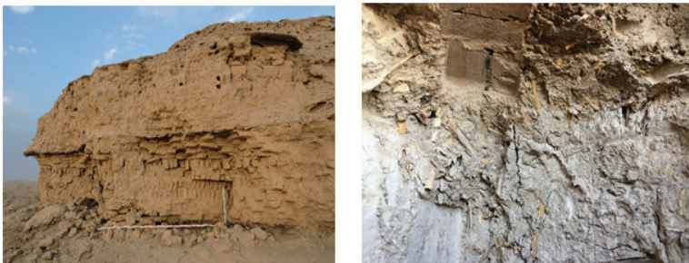
Figure 4a and b. Uruk, Eanna Ziggurat west corner before conservation work (a) and yellow straw in the mortar of the existing fabric (b)
