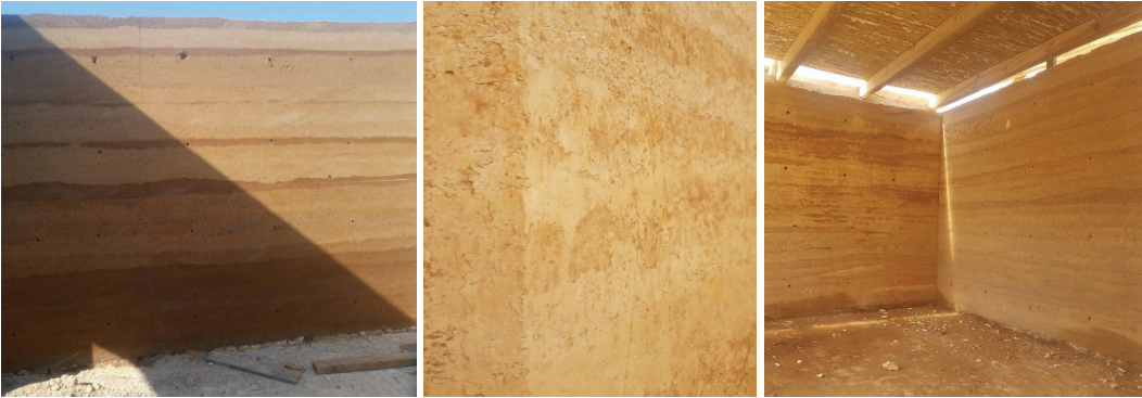
Figure 13. Various textures of rammed earth walls
