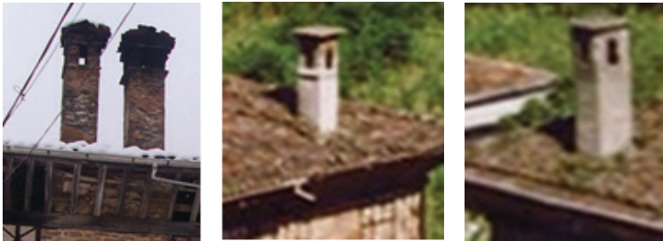
Figure 13. Balekoğlu Mansion Chimney Detail [F: E. Balık, 2019]
