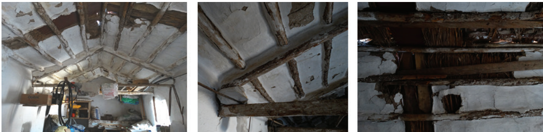
Figure 11 Interior view of wooden roof structure with ‘tartma’ beams and rafters (2018).
