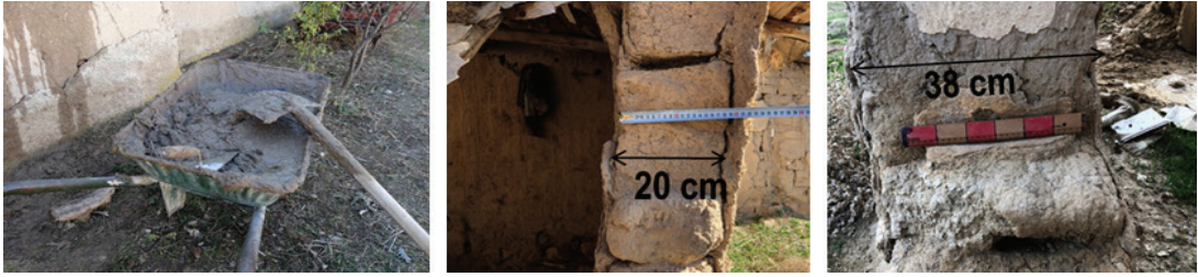
Figure 7. Sludge made of ‘barren soil’, fine straw and water mixture (2018).
