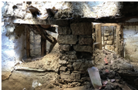
Figure 3 a. Rear wall made from stone
