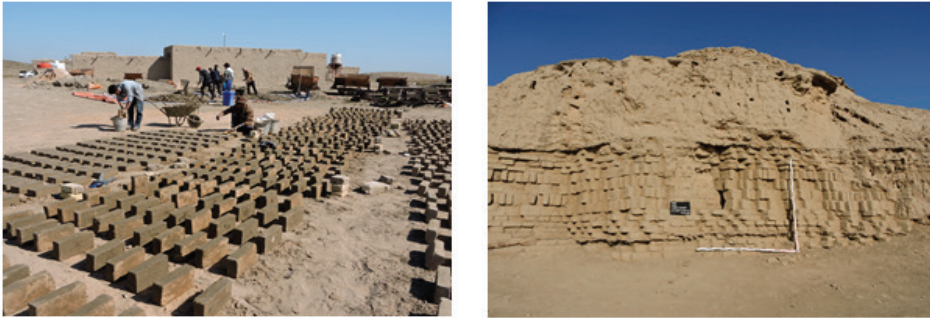
Figure 5a and b. Making earth blocks in the traditional method (a) and a view of the western corner of Eanna Ziggurat after completion of conservation work (b) in 2019
