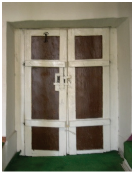
Back elevation photo
