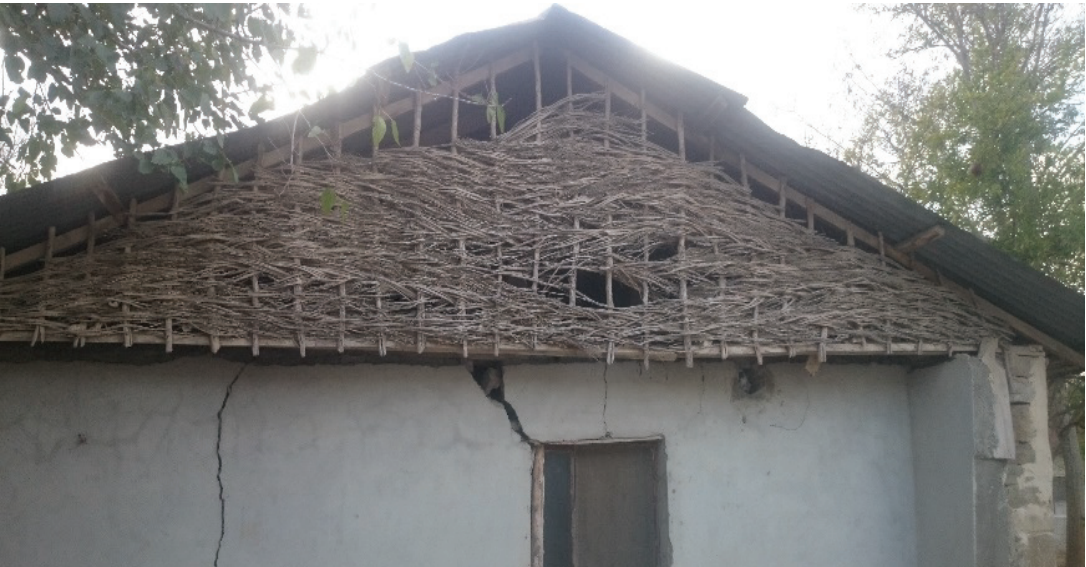
Figure 14: View of Muhacir Houses Roof [2]
