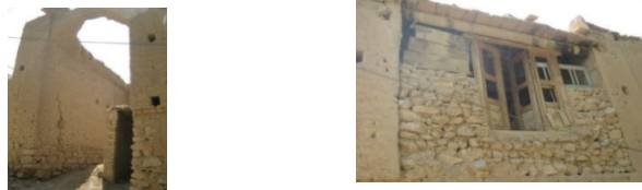
Figure 4 and 5. From left to right: the corridor near the entrance - first floor rooms
