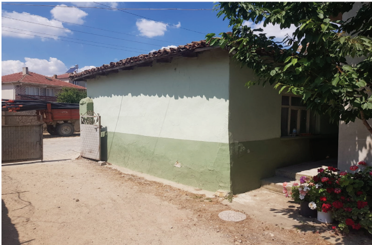
Figure 4. Sample mudbrick housing garden entrance
