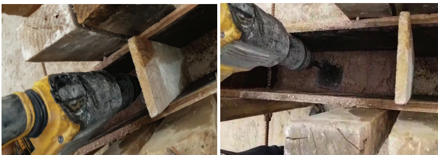
Figure 6. Using the drills as a compactor with apparatuses (Photo Credit by, Author)
