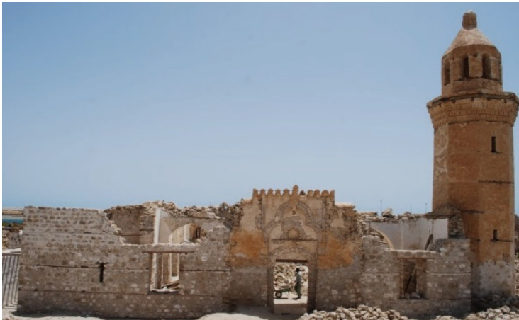
Figure 11. Shafii mosque main elevation
