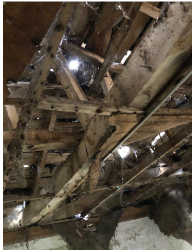
Figure 8. Purlin and poles related to the roof structure
