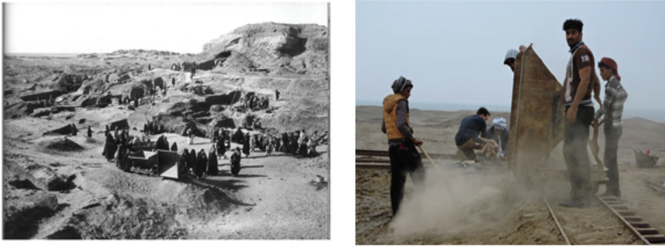
Figure 3a and b. The railway during excavations (a) (1923) and during reactivation (b) in 2018
