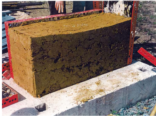
Resim 3.1. Şantiyede Dökölen Numune Blok Picture 3.1. Sample Block Casted in Construction Site
