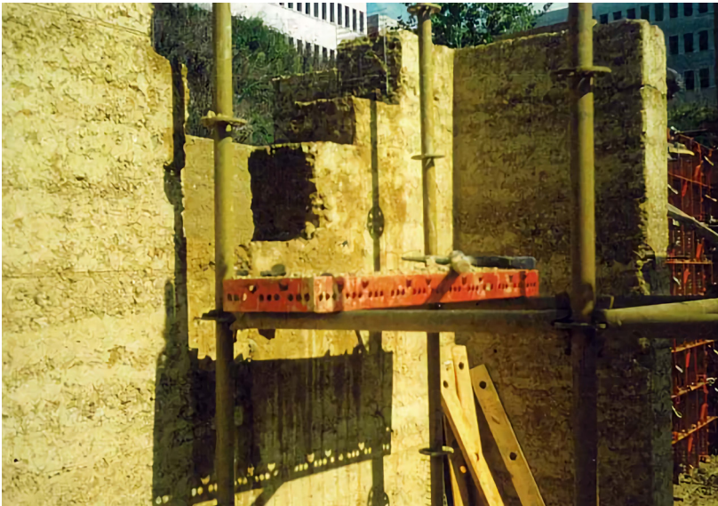
Resim 3.24. Hatalı İş Derzinin Onarılması Picture 3.24. Repair of Defected Construction Joint
