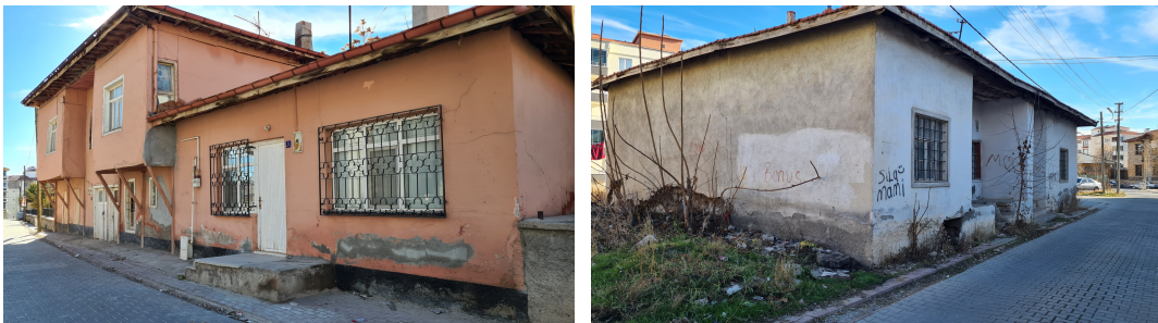
Figure 6. Change in frame material, damage caused by paint and inscriptions on the facade (Author's Archive)
