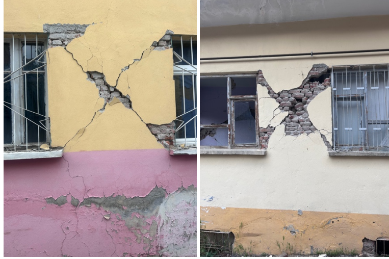
Figure 11. Examples of structural cracks [11]
