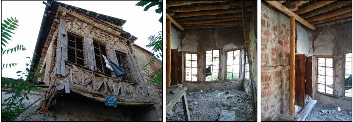
Figure 15. Structural damages observed in the interior and exterior parts of the bay window on the eastern façade of Faik Bey Mansion (2023)
