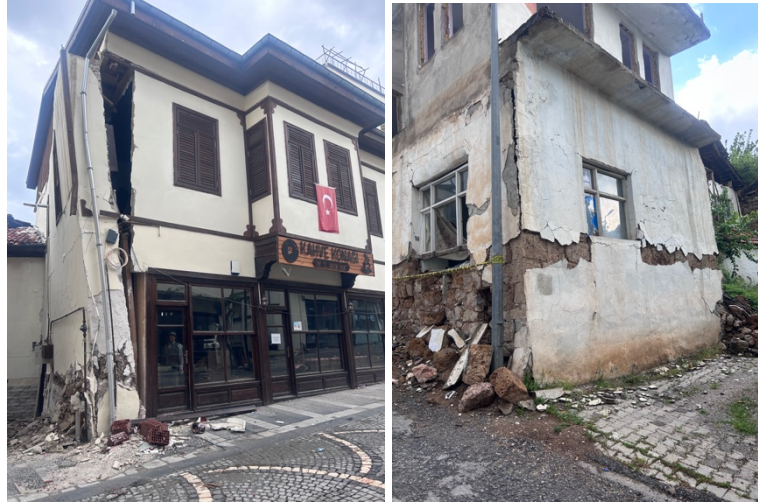
Figure 13. Examples of damage to the corner [11]
