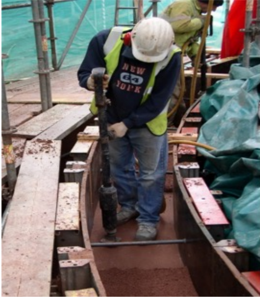
Figure 2: Compression technique
