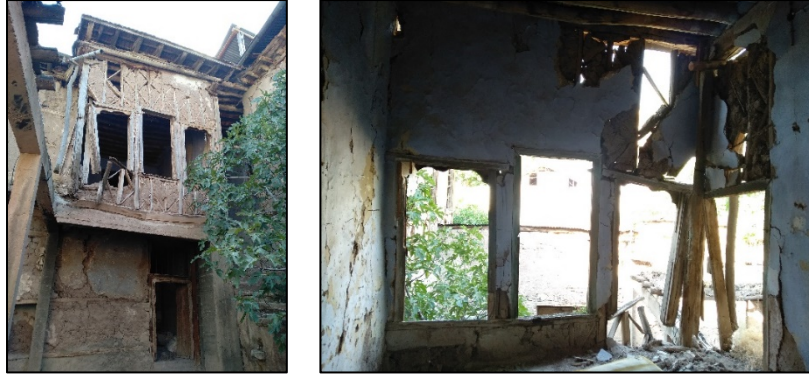
Figure 16. Structural damage observed in the bay window of the hall facing the courtyard of Faik Bey Mansion (2023)
