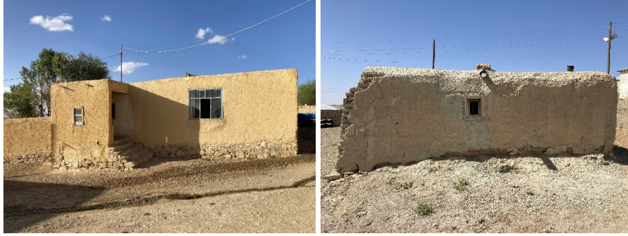
Figure 5. Examples of adobe houses from the village of Mollatopuz in Van (Gökdemir Archive)
