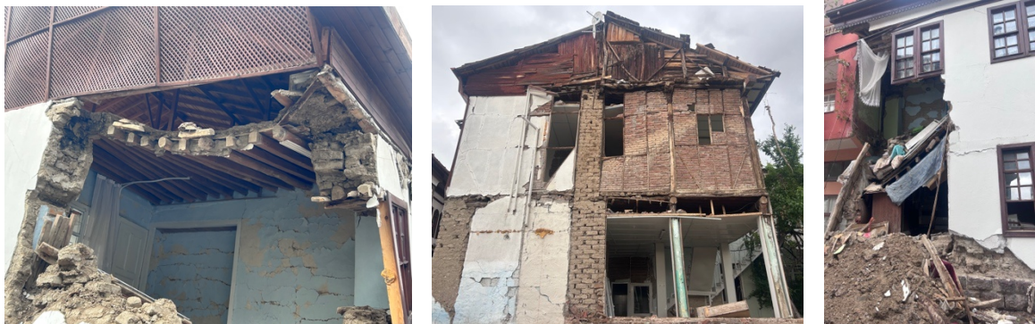
Figure 8. Examples of collapse due to ceiling load [11]
