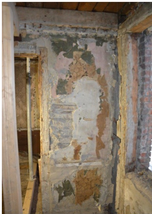
Figure 3. Traditional type of vernacular Nordic timber and earthen construction (earth mortar layer between squared timber in wood framing) with “rapping” (a type of Norwegian clay plaster on wooden surfaces), in the house Smedbakken 5 from 1845/46 in Trondheim, Norway (source: author)
