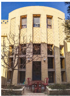
Figure 28. South facade rotation and the placement of windows in the great wall depth
