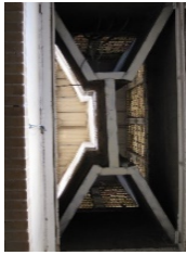
Figure 13. Internal partitions of Windcatcher
