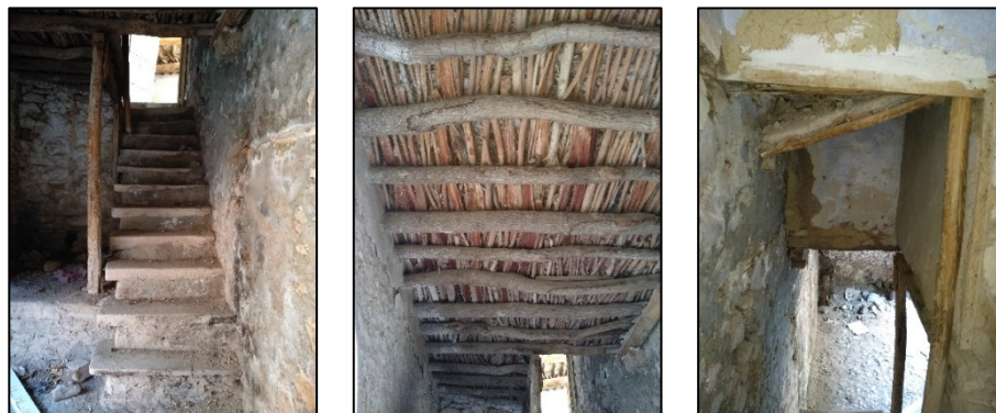
Figure 12. Damages observed on the stairs and ceiling tiles in the iwan section of Faik Bey Mansion (2023)
