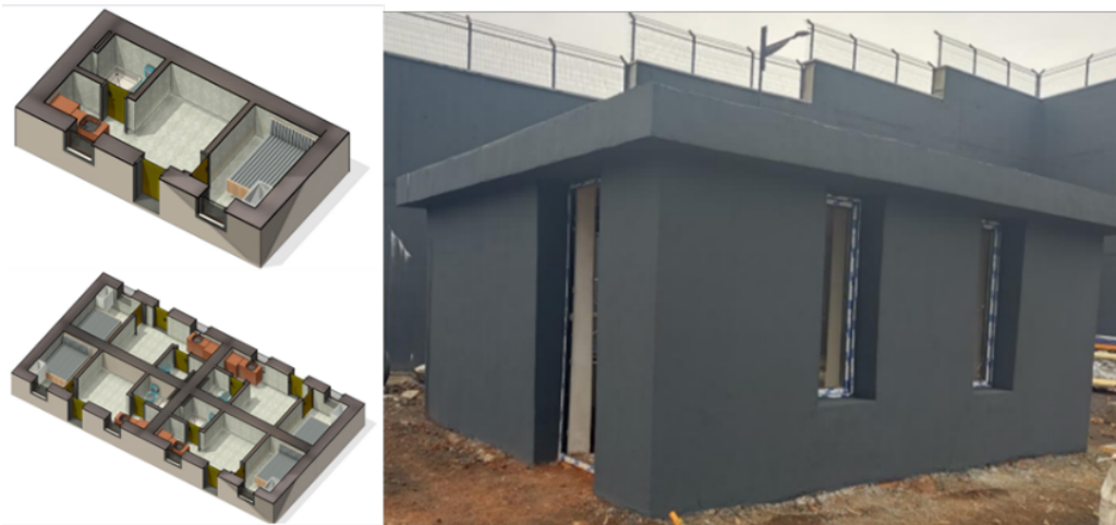
Figure 5: Temporary shelter plan produced from earth, 4-module system and the final version of the temporary shelter
