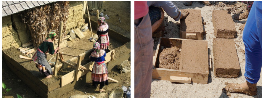
Figure 5. Earthen Construction Techniques [11].
