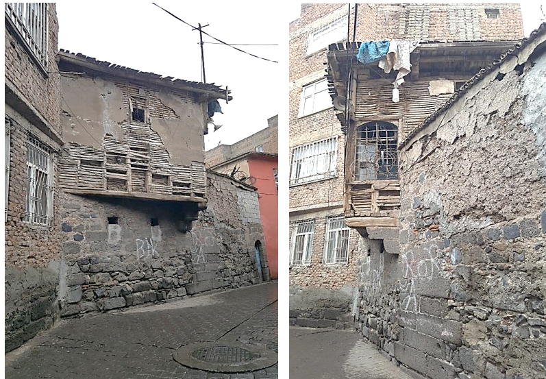
Picture1. A bay window made with the bagdadi construction technique in the Suriçi region of Diyarbakır
