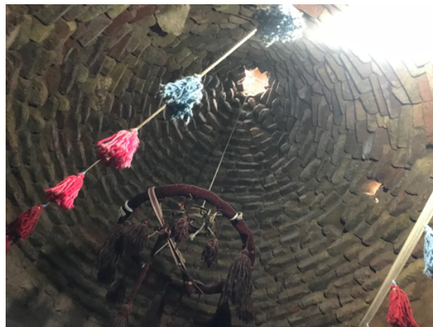
Figure 4. The longitudinal section of the dome has developed in a parabolic/conical shape (Photo by authors)
