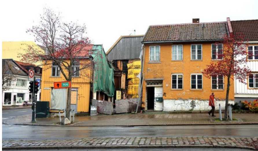
Figure 1. The façade of Smedbakken 5 in Trondheim built in 1846: approx. 40-year-old paint that acts as a vapour barrier and visible damage to the building physics caused by disturbed micro-meteorology: frost wedging, cracks and flaking of the paint (source: Adresseavisen)
