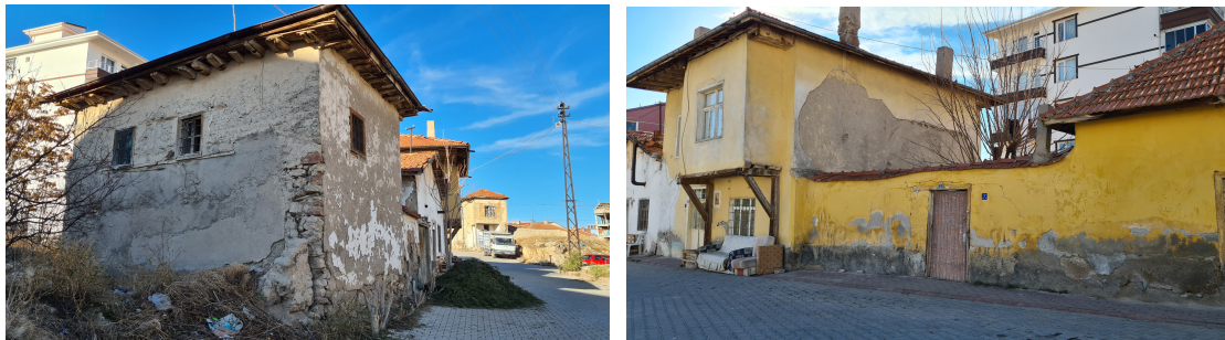
Figure 4. Erosion and plaster repairs on body walls (Author's Archive)
