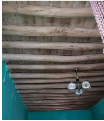
Fig.3.7. Beaming system (cisir) in Hüseyinik houses
