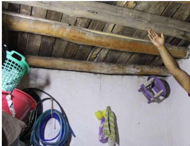
Figure 3. Issues like 'cracks and deformations, fungal and pest damage, warping and bending, and color changes' observed in the flooring of an adobe house in Şırnak are due to temperature variations.
