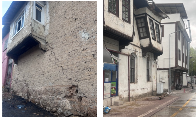
Figure 7. Examples of separation of the annex [11]
