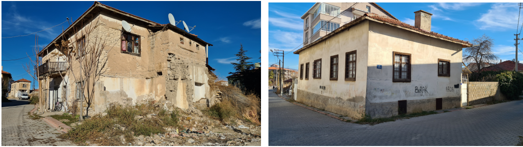
Figure 5. Later added spaces and application of concrete plaster (Author's Archive)
